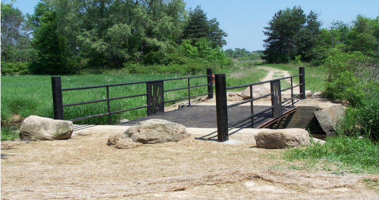
Shiawassee Pathways Trail Under Construction (2010)
