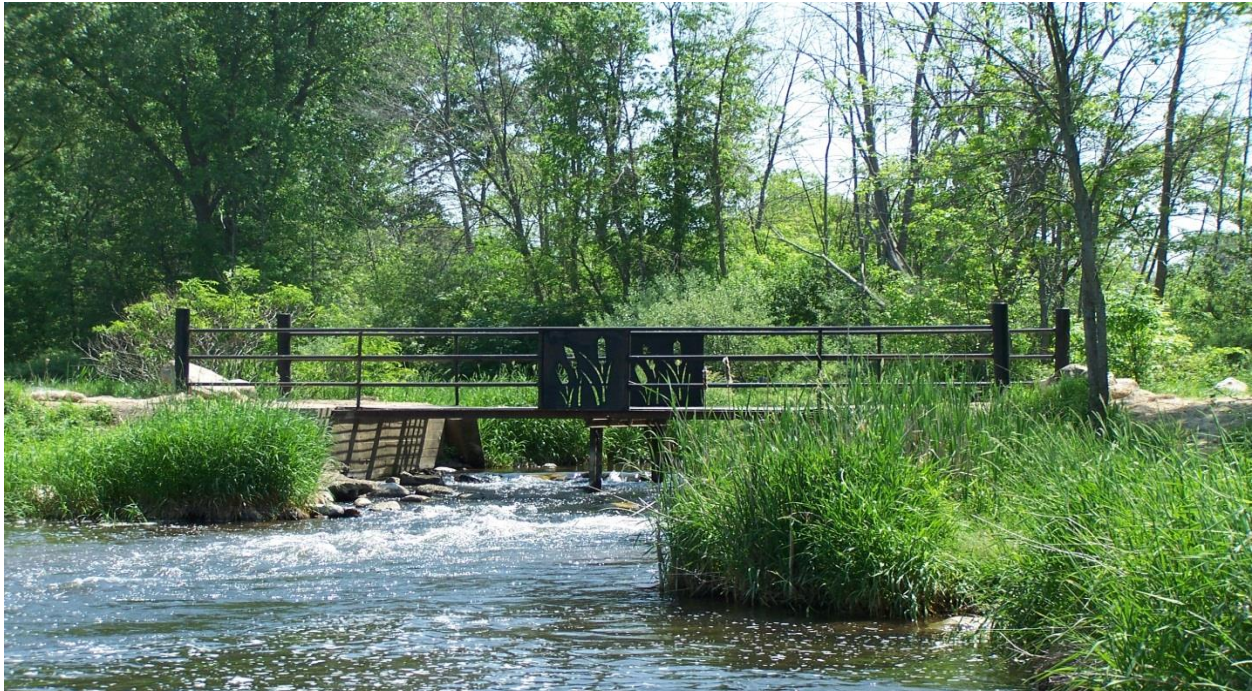
Bridge at The Shiawassee Pathways
