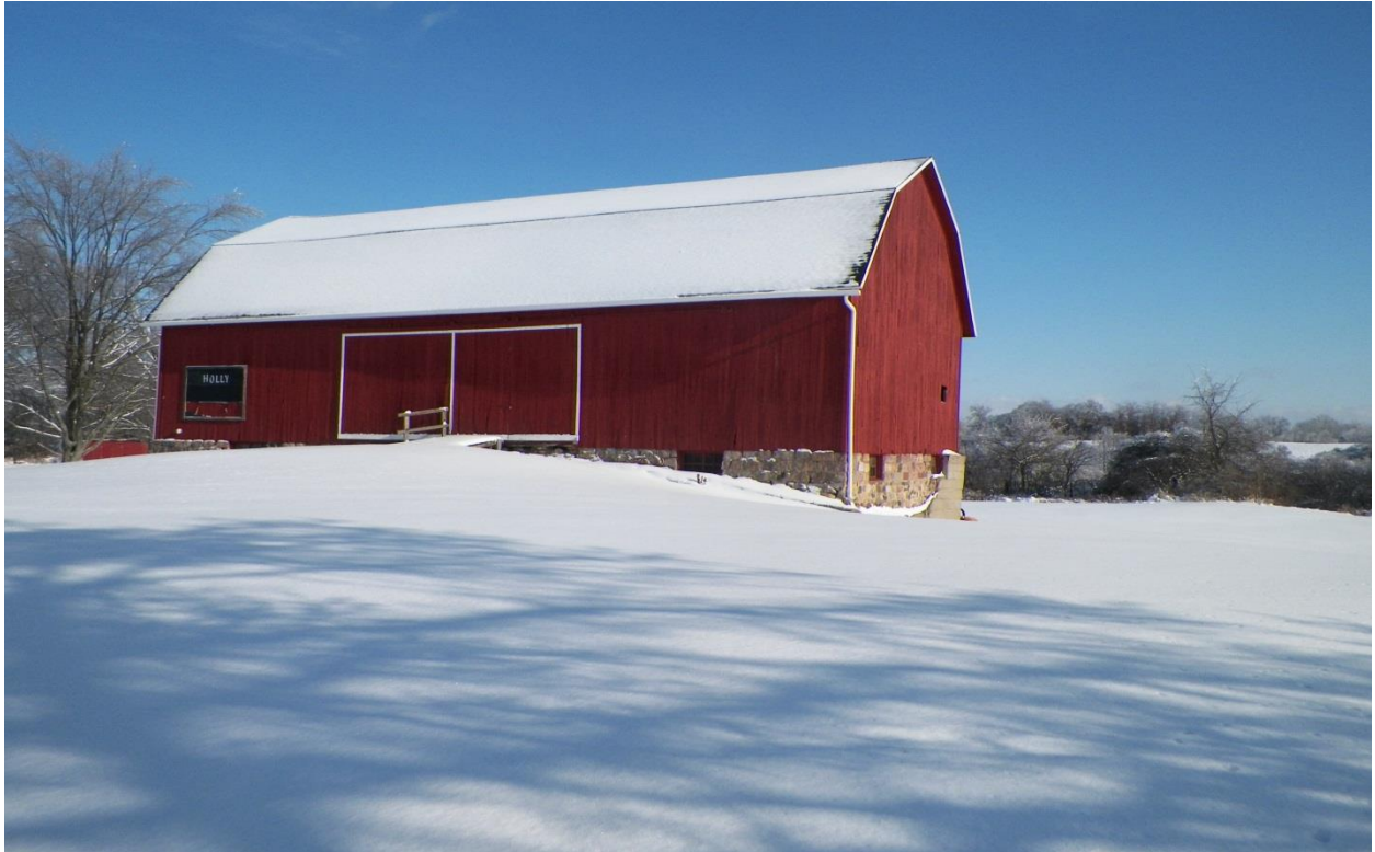
Post and Beam Barn at Holly Farmstead
