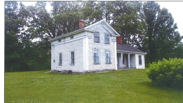
Figure 4: South House, photo by Ron Campbell, June 2018
